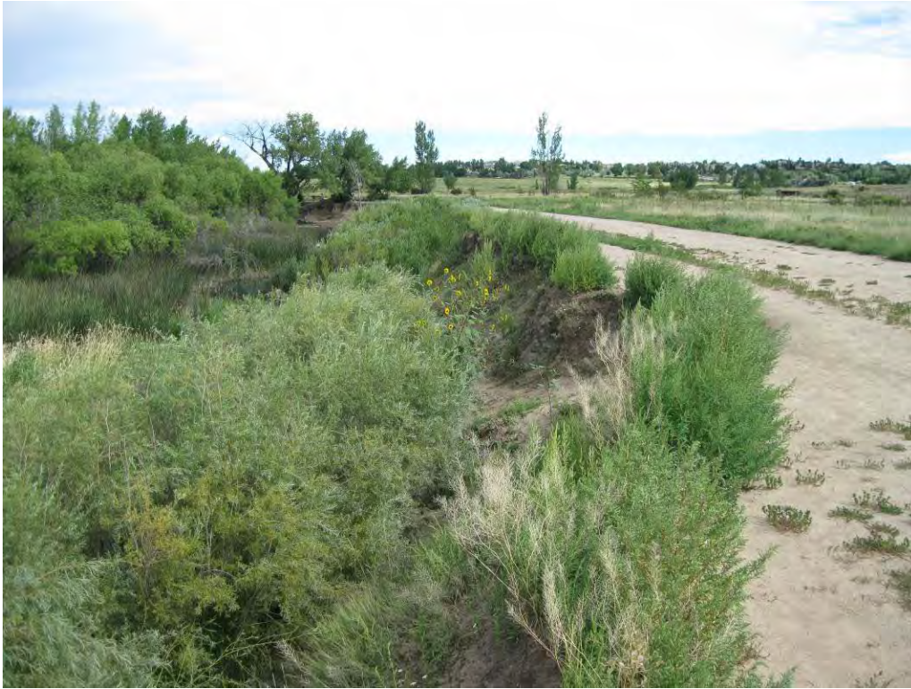
EXHIBIT 1-2 Reach 1: Upstream Reach Cherry Creek Stream Reclamation at 12-Mile Park Project
