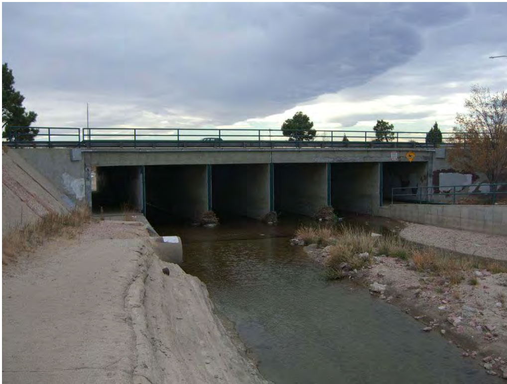
EXHIBIT 4-3 Example of Soil Cement – Sand Creek, Colorado Springs, Colorado Cherry Creek at 12-Mile Park Alternatives Analysis
