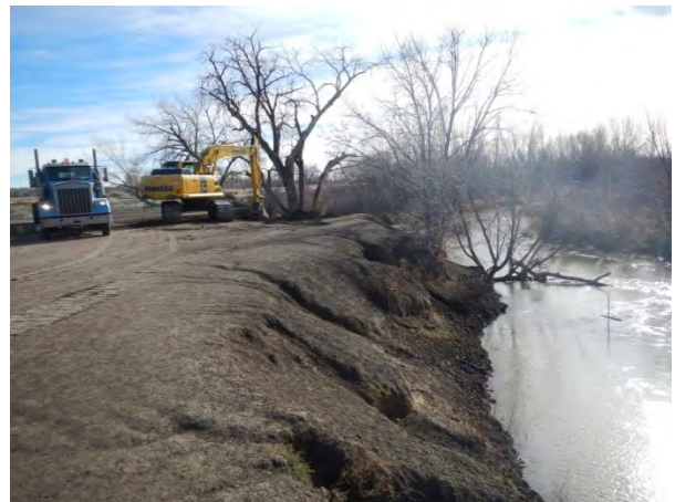
Photo 6: Tree extending from bank (December, 2013)
