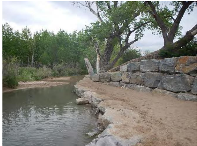
Photo 7 - Access Beach @ Existing Tree
