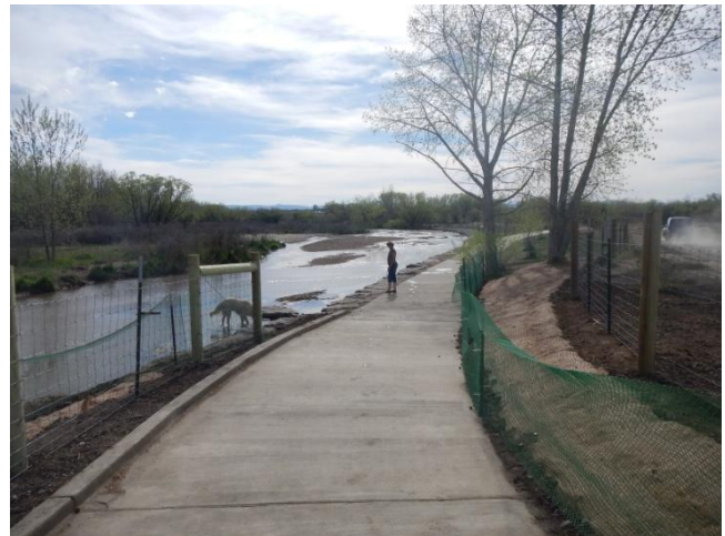
Photo 4 - Connection with the Phase I Project
