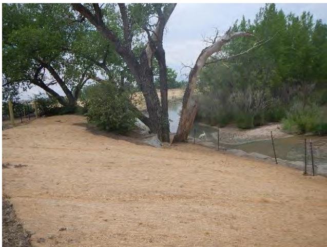
Photo 10 - Stabilized Slope (seeded & blanketed)
