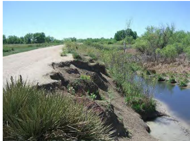
Photo 1 - Steep Creek Banks
