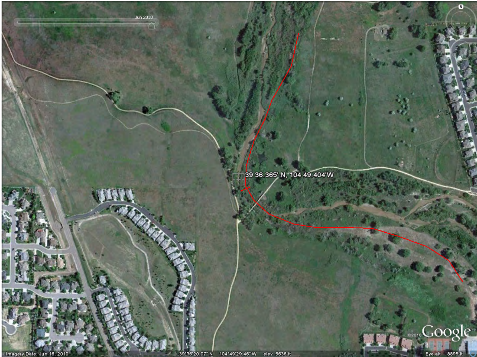
Figure 7. June 2010, Aerial Photograph of Site #1
