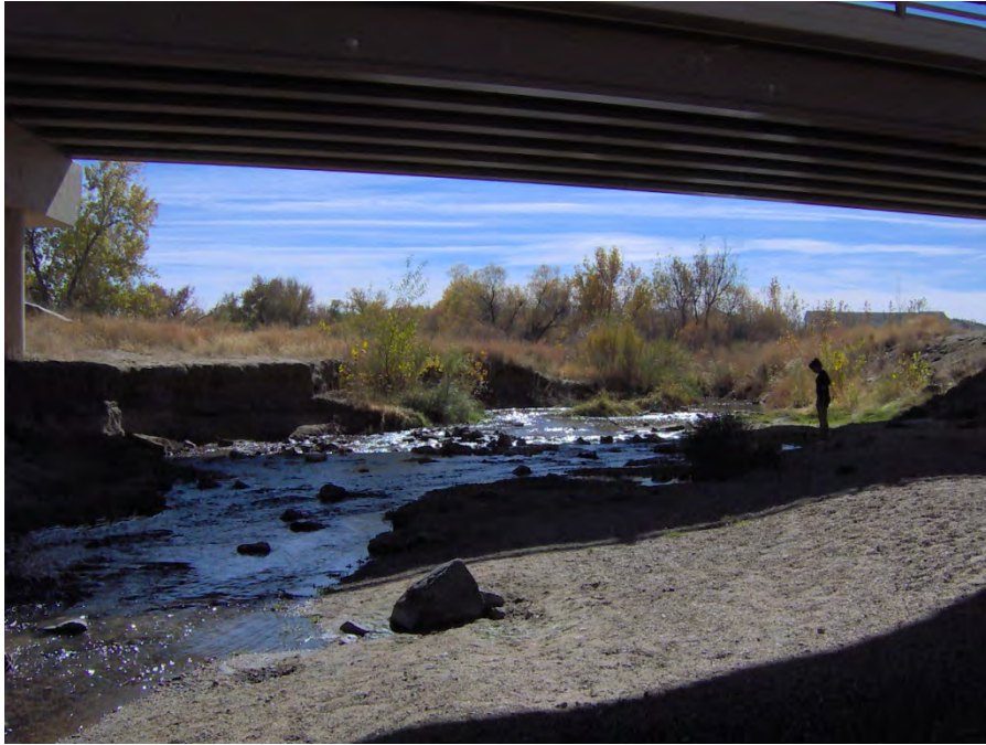
Figure 22. Site #4 – Stream bed material sample at Broncos Parkway
