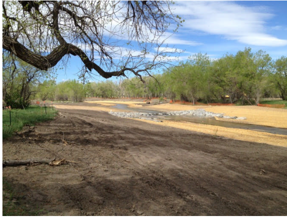
Photo 3 - Post project with side channel
