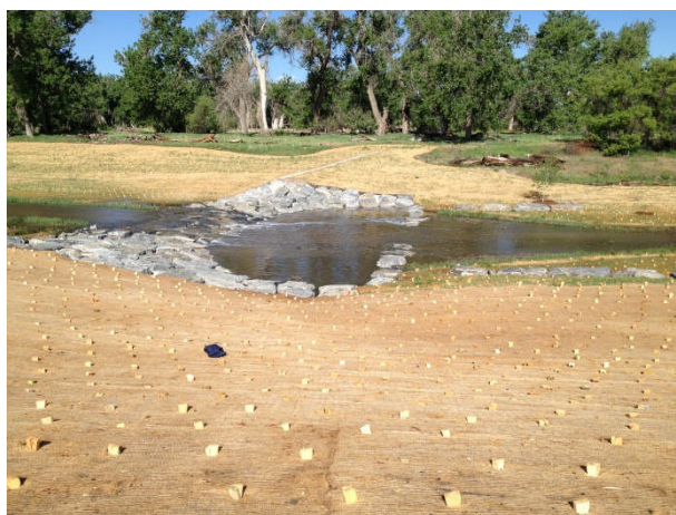
Photo 2 - Post project drop structure
