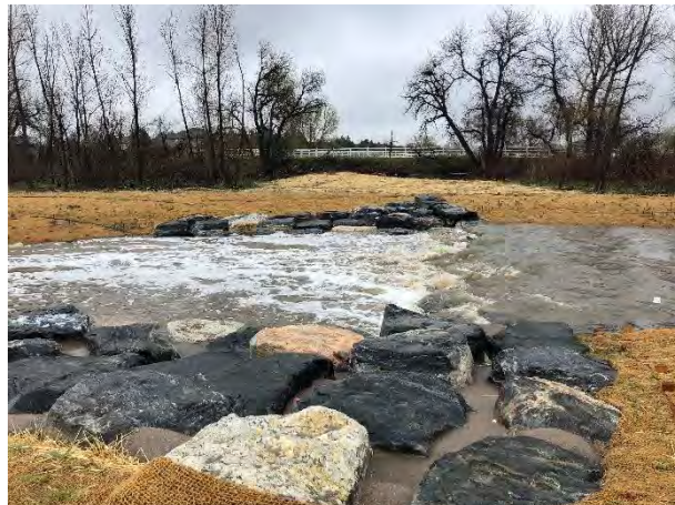
Photo 9 – Constructed Grouted Boulder Drop
