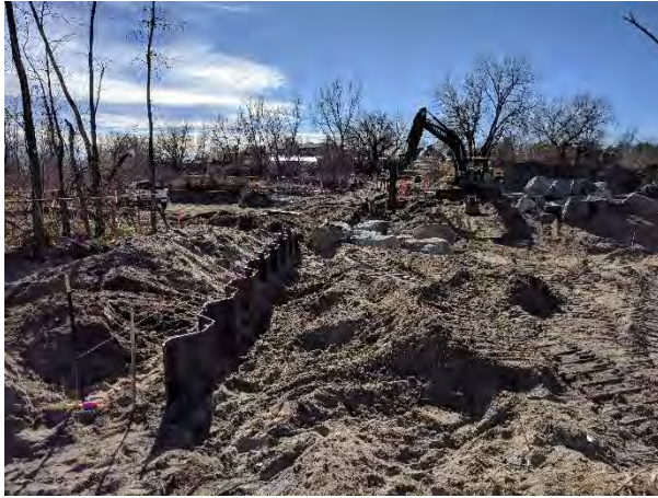
Photo 5 – Channel Grading
