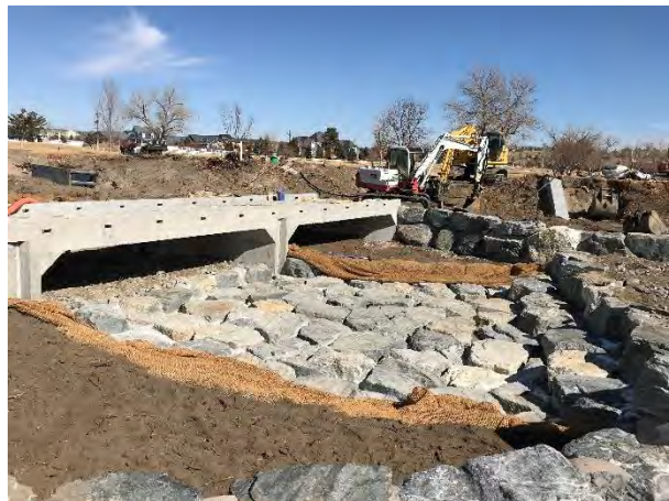
Photo 7 – Grouted Boulder Drop Construction
