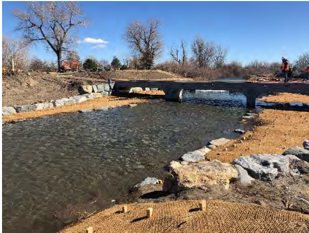
Photo 10 – Constructed Channel @ Golf Cart Bridge
