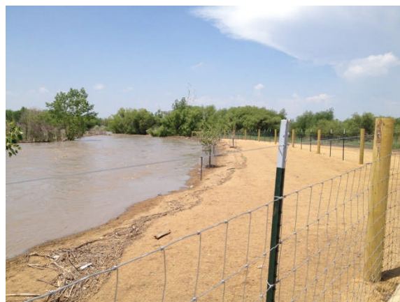
Photo 6 - Restored Breach Area
