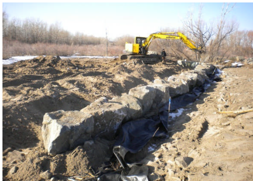
Photo 3 - Boulder Toe Wall
