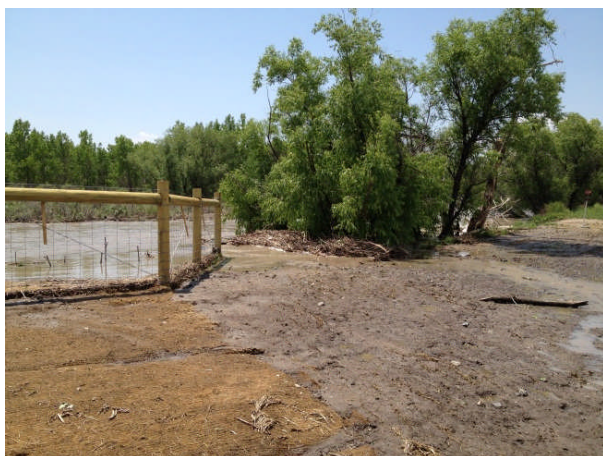
Photo 7 - Bank Overflow Area
