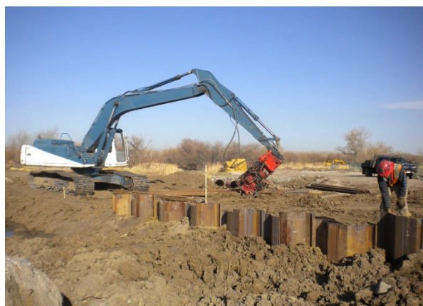
Photo 4 - Sheet Pile Cut-Off Wall
