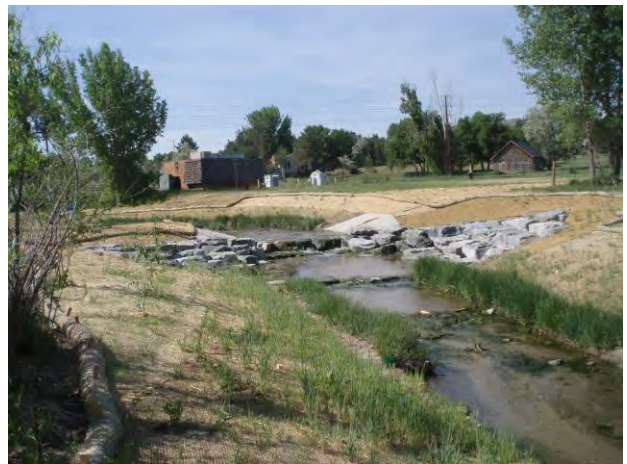
Photo 9 – Constructed Channel & Grouted Boulder Drop Structure
