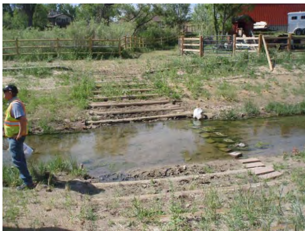
Photo 10 – Constructed Channel & Equestrian Crossing
