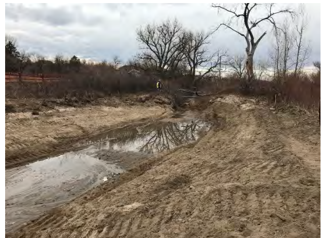
Photo 6 – Channel Grading
