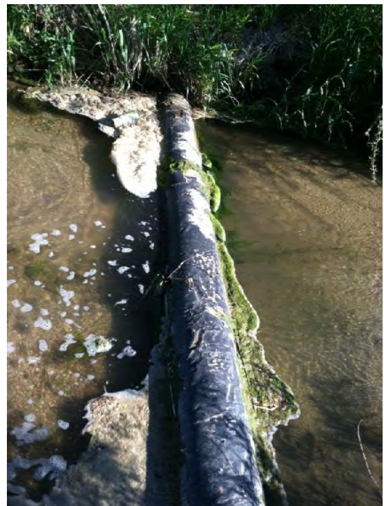
Figures 11 and 12. Aggradation on Floodplain Adjacent to Active Channel, and Undercut Pipeline Showing Evidence of Degradation in Active Channel (Muller)
