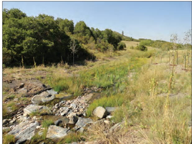
Photo 5b - View to the northwest of wetland vegetation establishing in the drop structure and channel bottom within the upstream portion of Reach B.
