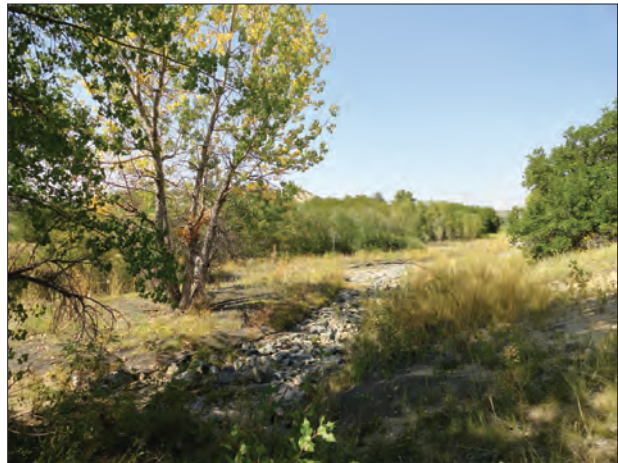
Photo 11b - View to the north of channel lining and vegetation along the channel banks at the upstream end of Reach C-lining.
