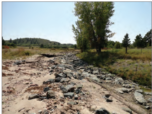
Photo 15b - View to the south of bank erosion and displaced riprap within the downstream portion of Reach E.
