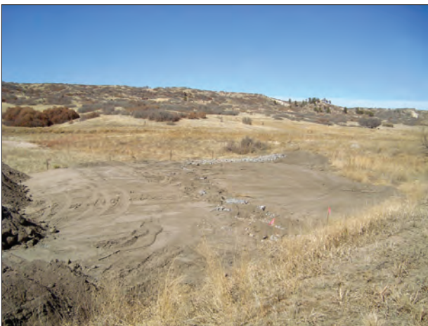
Photo 18a - View to the north during construction of the rundown structure within Reach G.
