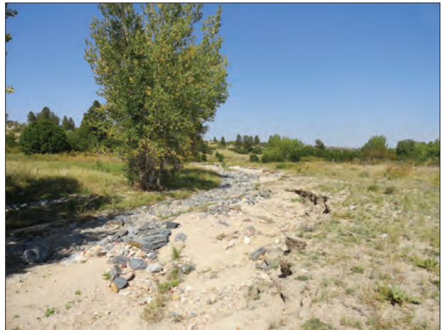
Photo 14b - View to the northwest of bank erosion and displaced riprap within the middle portion of Reach E.
