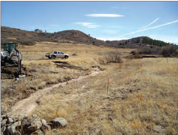
Photo 17a - View to the south during construction of the drop structure within Reach F.
