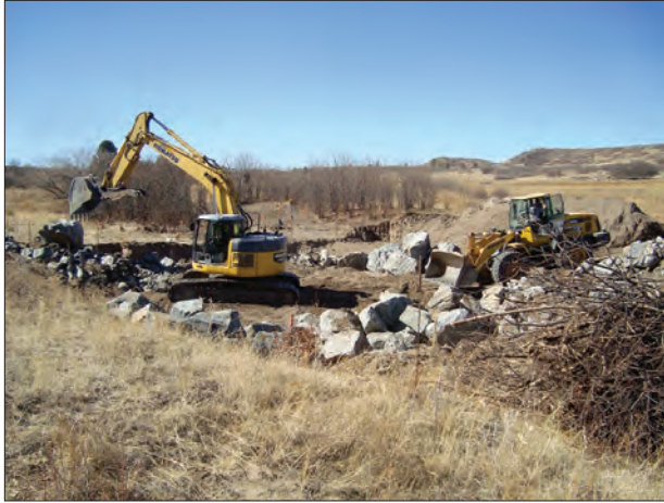
Photo 19a - View to the southwest during construction of the drop structure within Reach H.
