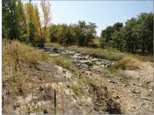
Photo 13b - View to the southwest of drop structure within the middle portion of Reach E.
