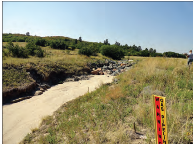
Photo 20b - View to the southeast of bank erosion and displaced boulders downstream of the drop structure at Reach I.
