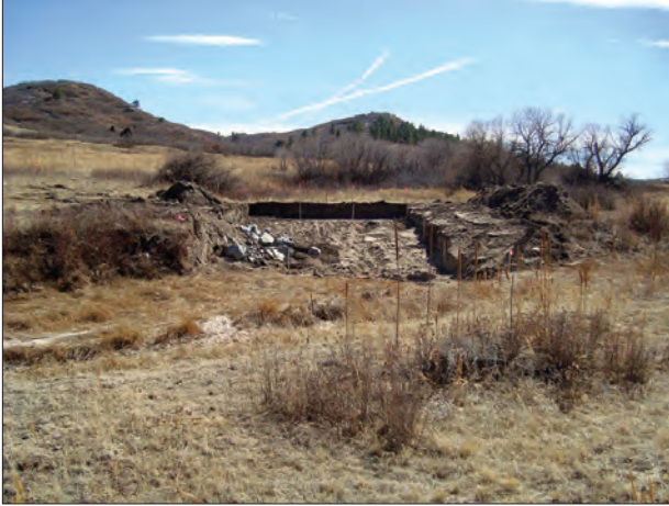
Photo 16a - View to the south of the rundown within Reach F during construction.
