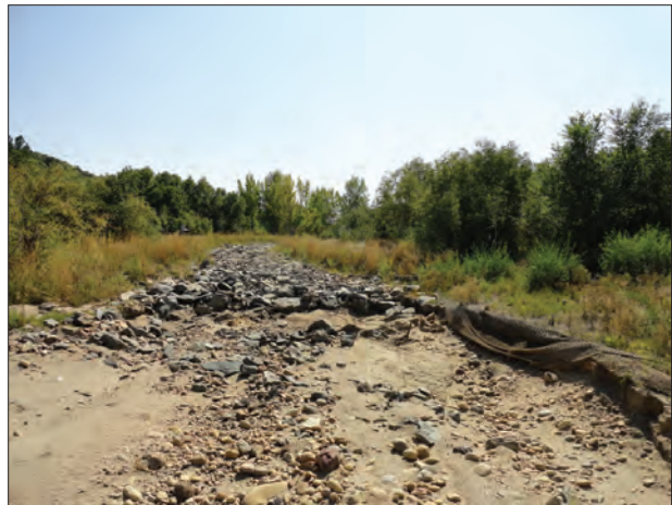
Photo 12b - View to the south of channel lining and displaced riprap at the downstream end of Reach C-lining.
