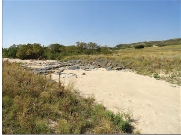
Photo 19b - View to the southeast of vegetation establishing in the uplands and sediment deposition within the drop structure and channel bottom at Reach H.
