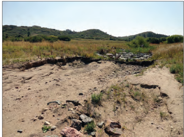
Photo 17b - View to the south of bank erosion and displaced riprap downstream of the drop structure at Reach F.
