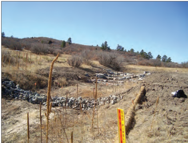
Photo 20a - View to the southwest during construction of the drop structure within Reach I.
