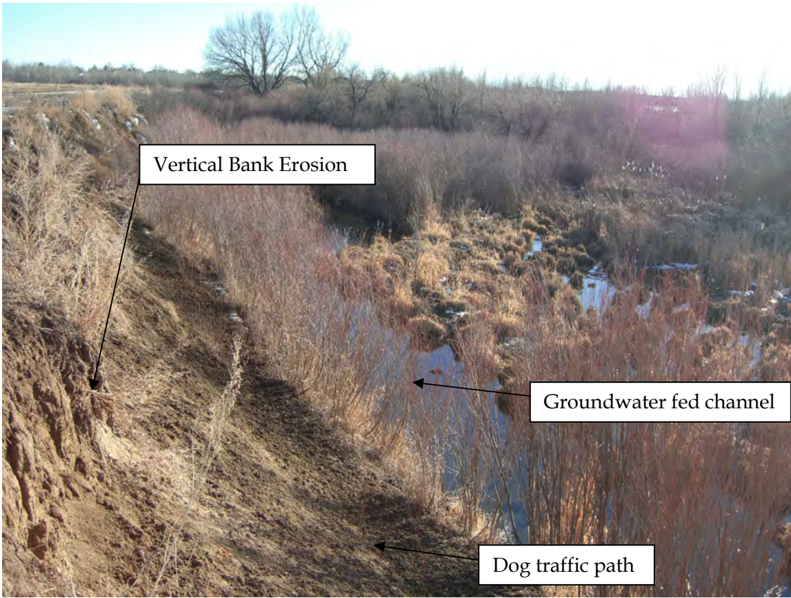
Photo 1 - Reach 1, Looking Upstream
