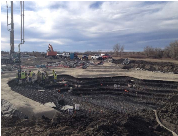
Photo 6 - Sculpted Concrete Drop Construction
