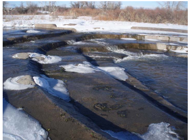
Photo 8 Constructed Sculpted Concrete Drop
