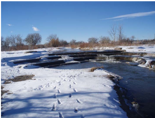
Photo 7 - Constructed Sculpted Concrete Drop
