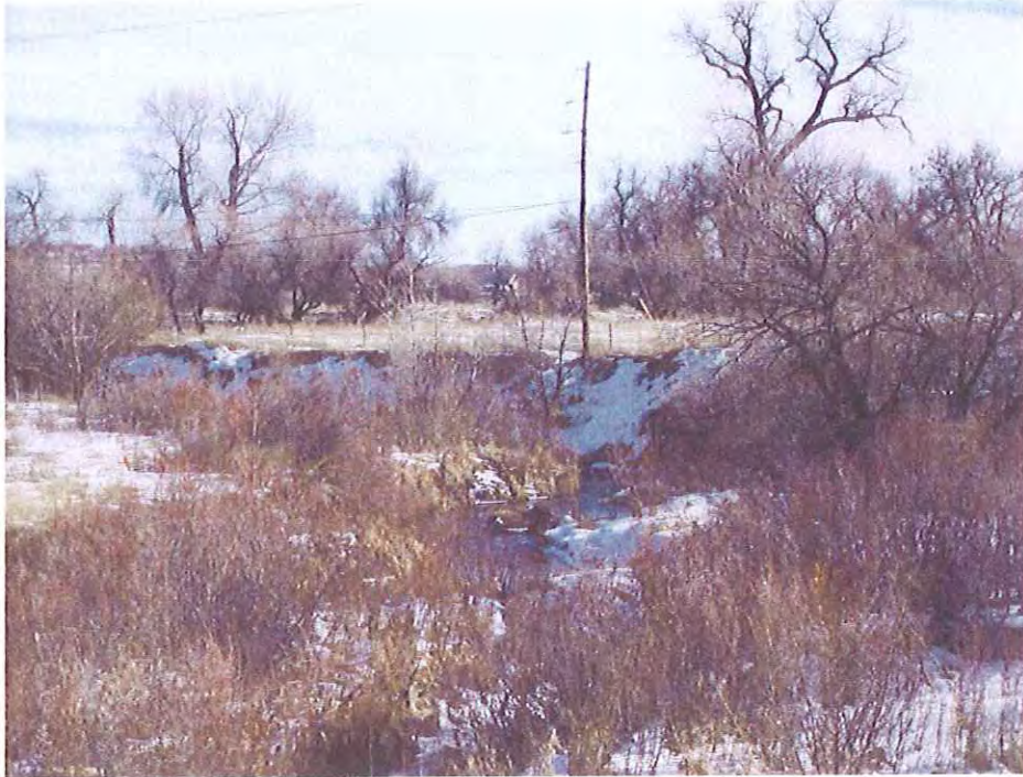
PHOTO 3 – CHERRY CREEK BANK EROSION UPSTREAM OF BRNCOS PARKWAY
