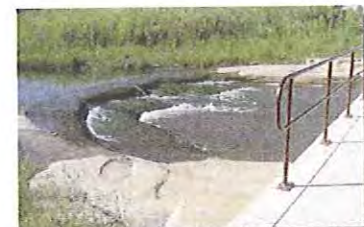
Trail Crossing and Drop Structure
