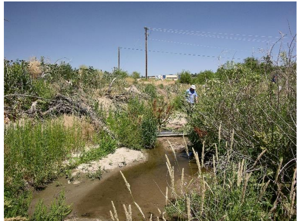
Photo 3 - Typical Pre-project Condition
