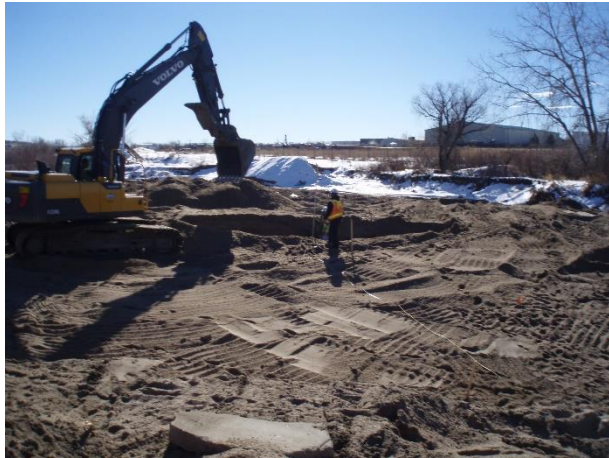
Photo 4 – Drop 14 Channel Grading
