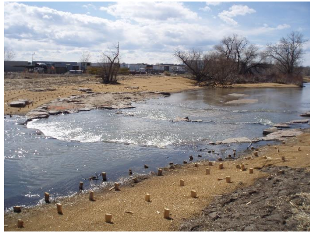
Photo 11 – Constructed Boulder Drop & Channel
