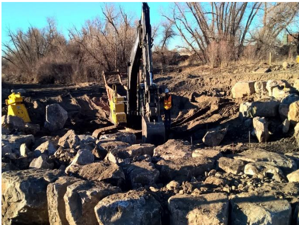
Photo 8 – Cascade Boulder Drop Construction
