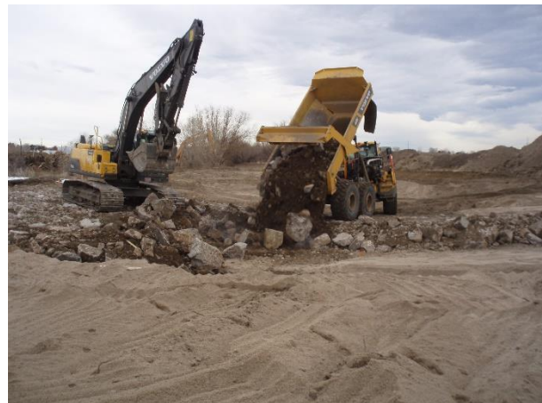
Photo 7 – Reach 5 Channel Construction
