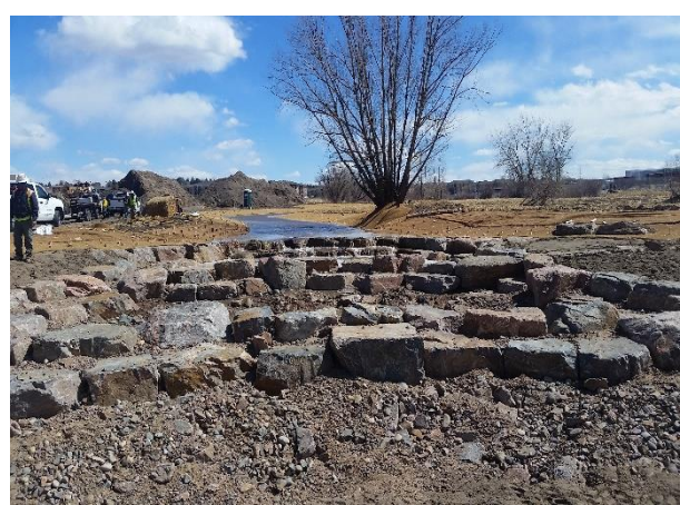
Photo 9 – Cascade Boulder Drop Construction
