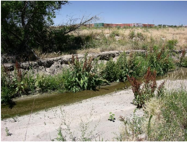
Photo 2 - Typical Pre-project Condition
