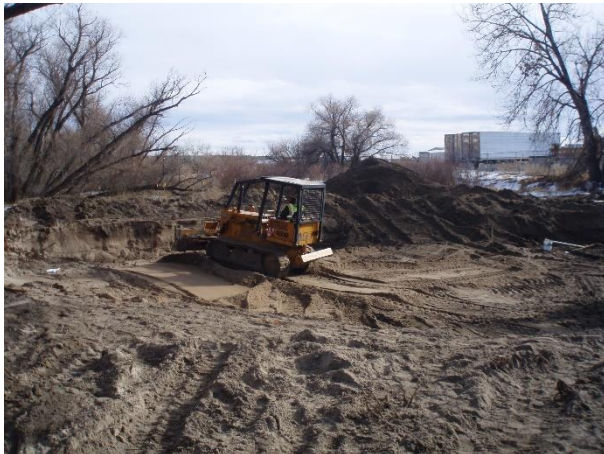
Photo 6 – Reach 5 Channel Grading
