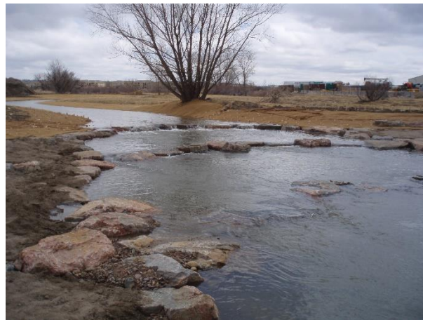
Photo 12 – Constructed Boulder Drop & Channel
