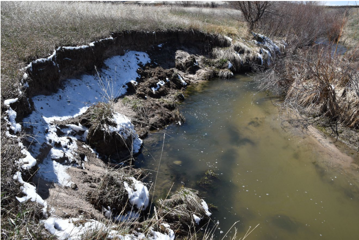
Figure 5: Existing Eroded Channel Bank (2020)
