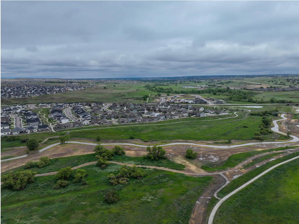
Figure 7: Central Portion of Cherry Creek Project Looking North (Courtesy of Naranjo Civil Constructors).
