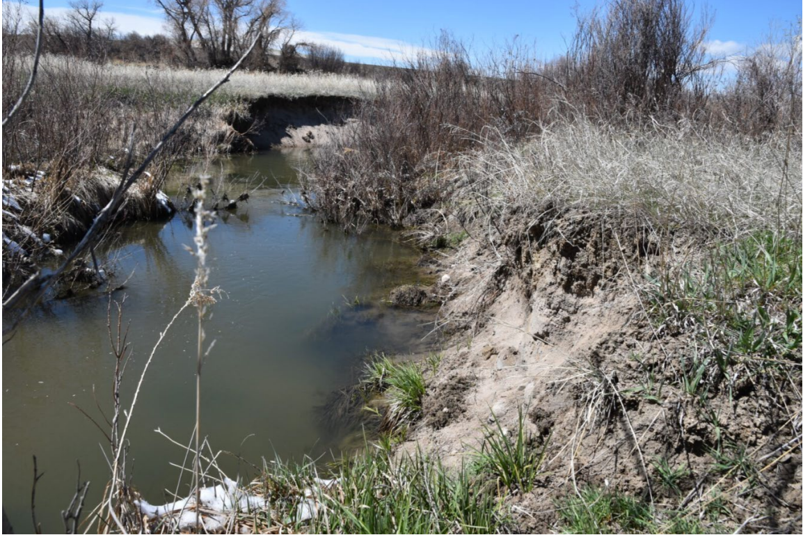
Figure 4: Existing Incised Channel (2020)
