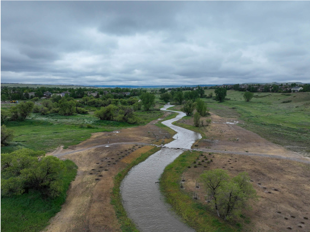
Figure 6: Cherry Creek Looking Downstream at Upstream Project Limits (Courtesy of Naranjo Civil Constructors)
