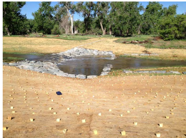
Photo 2 - Post project drop structure
