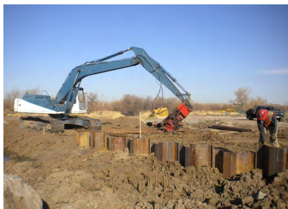
Photo 4 - Sheet Pile Cut-Off Wall
