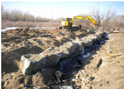
Photo 3 - Boulder Toe Wall
