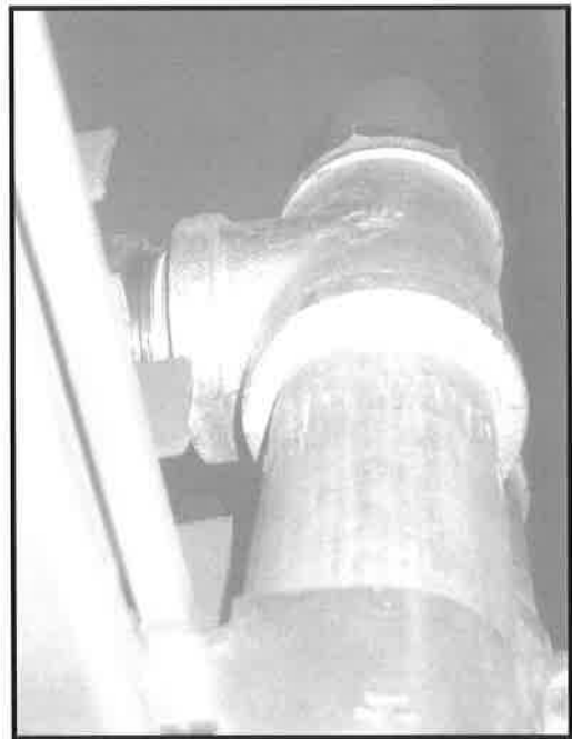
NEW BLOW-OFF SILENCER TYPICAL OF (4) FOUR
