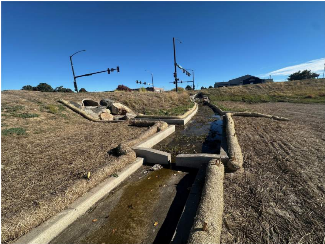
Figure 4: Concrete forebay at Northeast Pond Inflow
