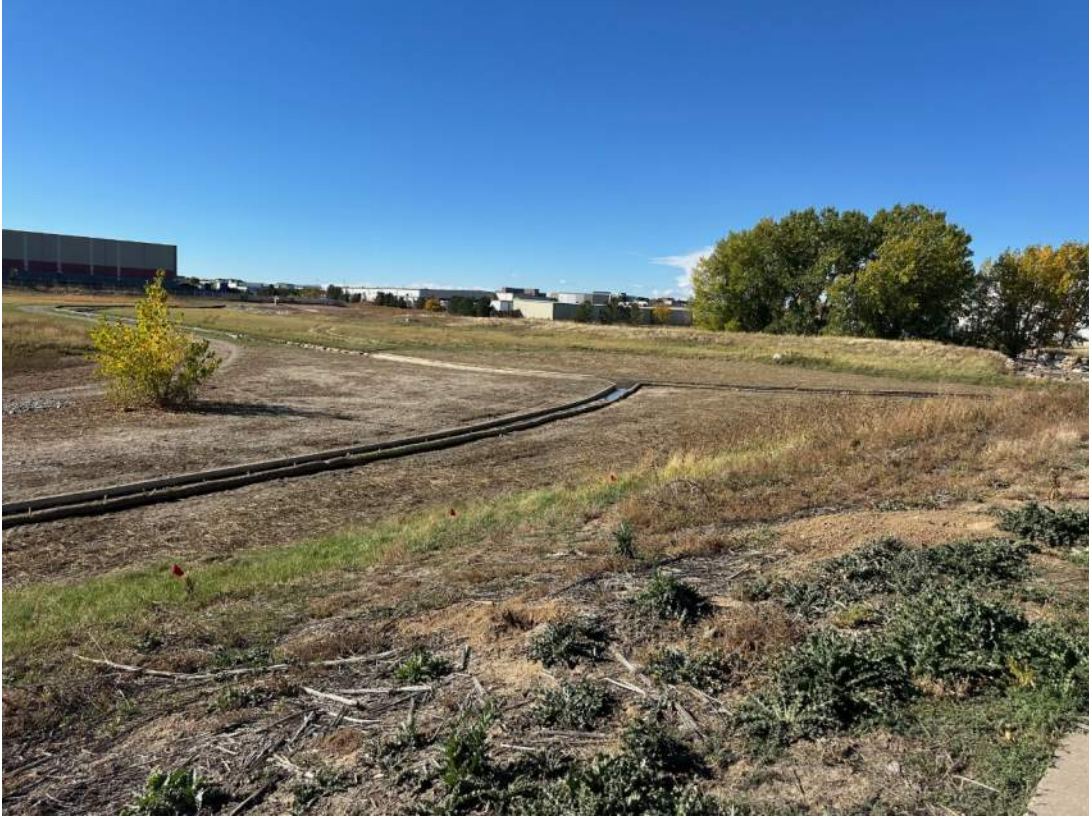
Figure 5: Overall Pond Completed with Maintenance Access
