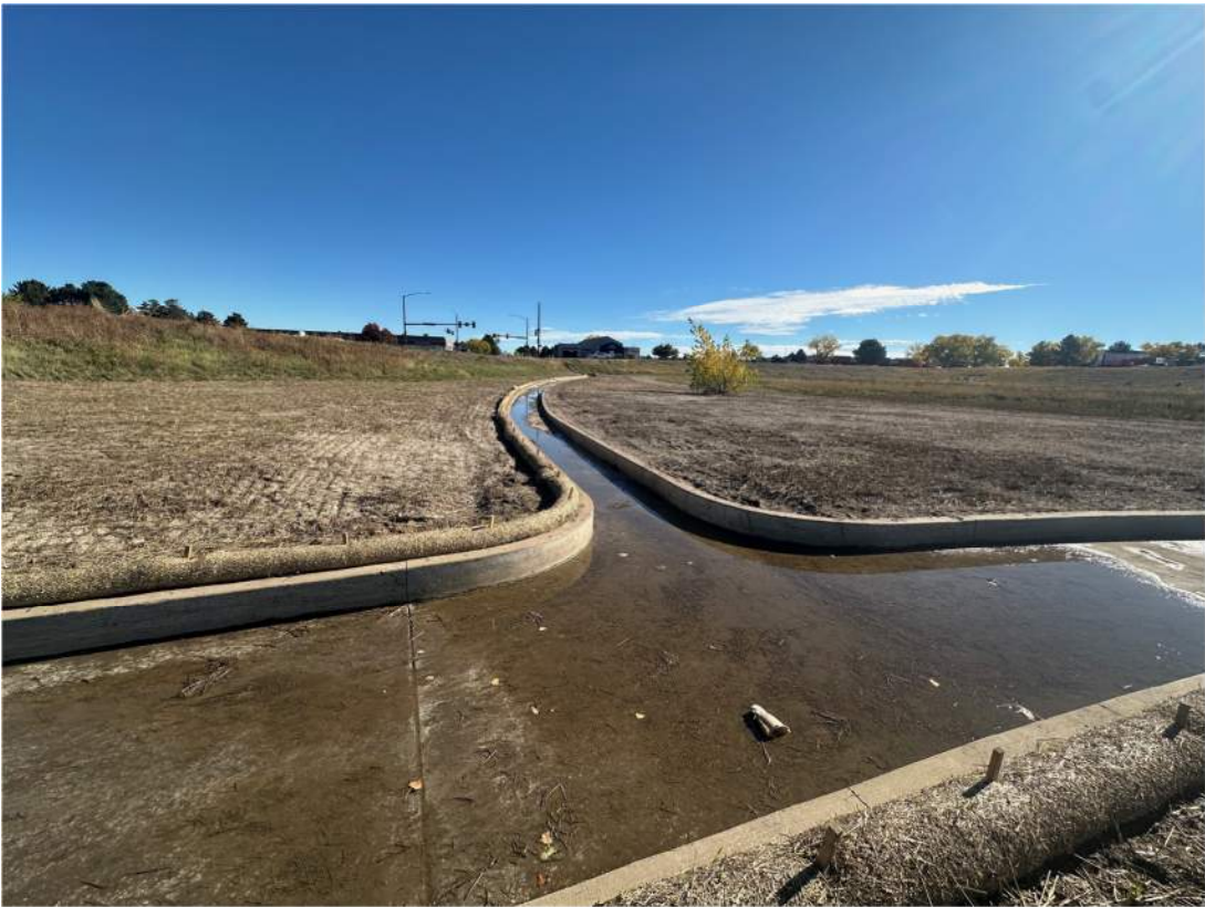
Figure 6: New Concrete Trickle Channel
