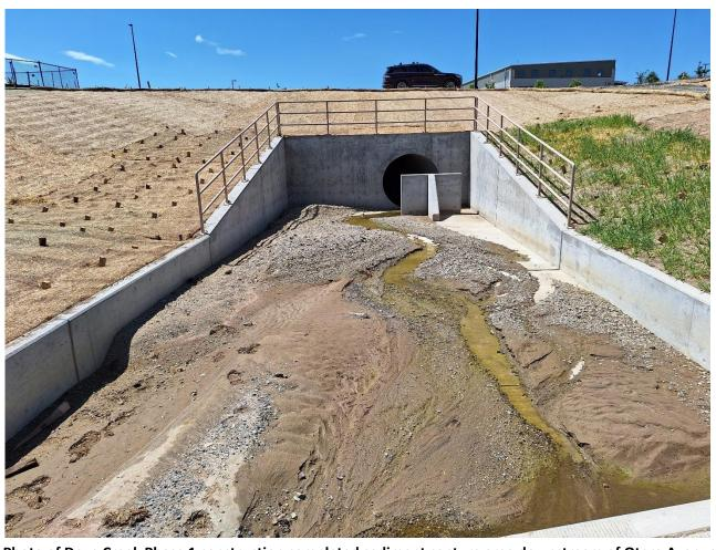
Photo of Dove Creek Phase 1 construction completed sediment capture area downstream of Otero Avenue
