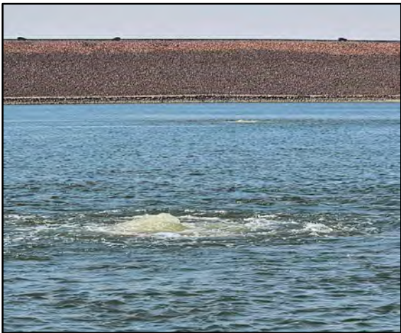
Two broken aerator heads showing overly vigorous aeration plumes
