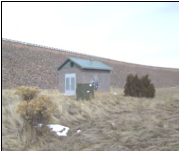
Compressor Building – Southwest of the Marina
