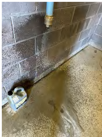
Photos showing accumulated water blown off and the compressor at "off" status
