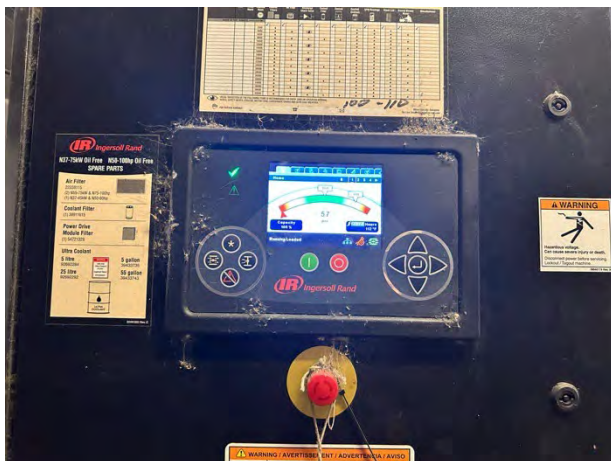
Compressor showing only 57 psi
