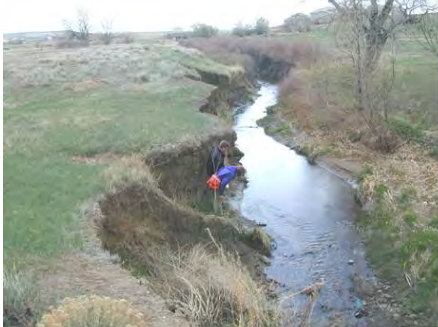
Figure 5-1. Cottonwood Creek Stream Reclamation - Before
