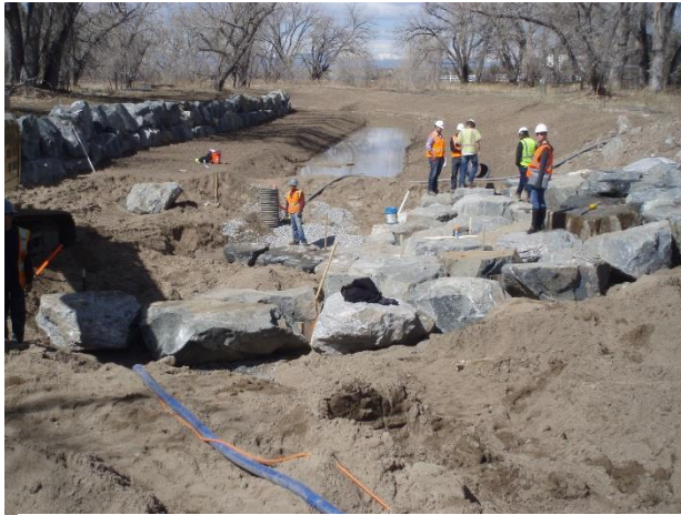
Photo 6 – Boulder Drop Structure Construction
