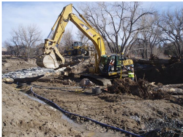
Photo 5 – Channel & Boulder Drop Construction
