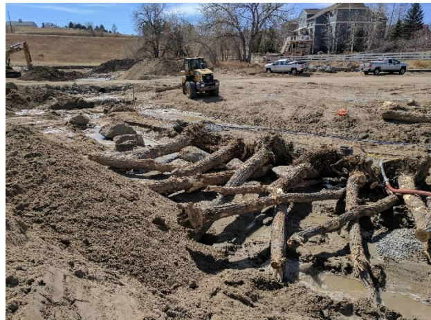
Photo 4 – Root Wad Stream Bank Protection Installation
