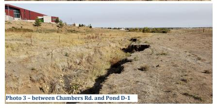
practice. RESPEC used step pool structures for grade control, bank protection (Void Filled Riprap, Soil Lifts, and Vegetation), and grading to create overbanks providing a wider stream corridor which stabilizes the stream and reduces erosion potential. The Project includes stream reclamation of approximately 2,700 linear feet.
