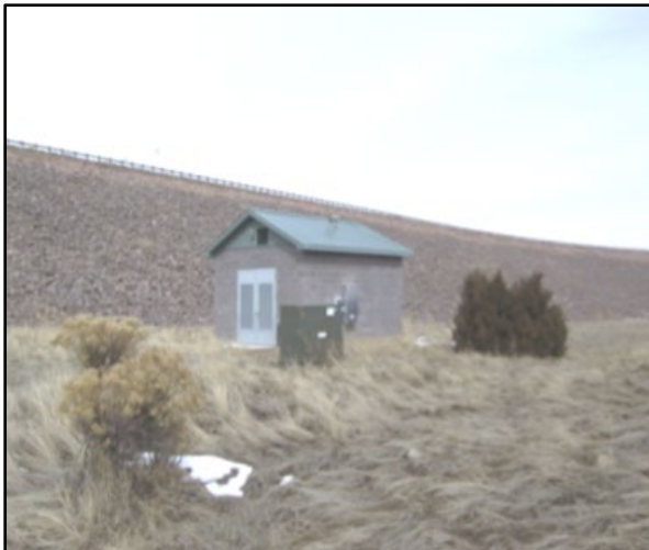
Compressor Building – Southwest of the Marina
