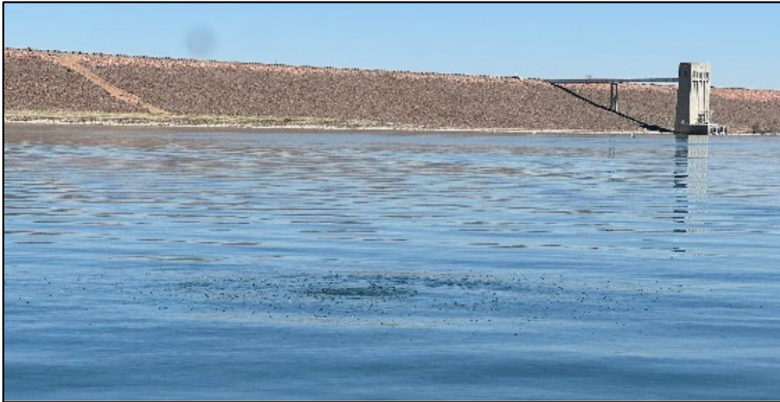
Normal aeration plume appearing as bubbles distributed on the water surface.
