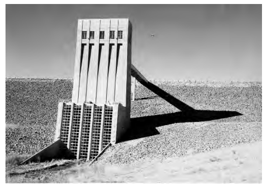
CHERRY CREEK DAM - 20 November 1951 Upstream face of Intake/ Control Tower showing trash racks.
