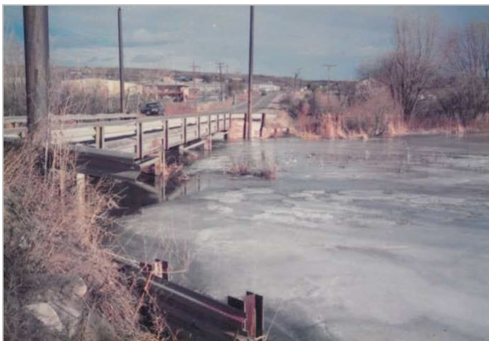
Figure 6-18. Titan Road Bridge over Plum Creek
