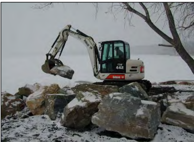
PRF maintenance at Dixon Grove.
