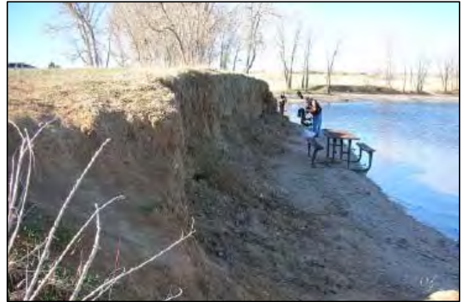
Example of shoreline erosion at Mountain and Lake Loop Trails
