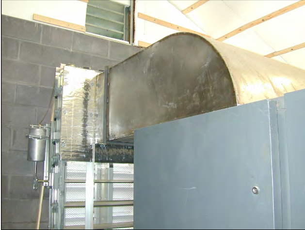
Improvements to compressor building for destratification system.
