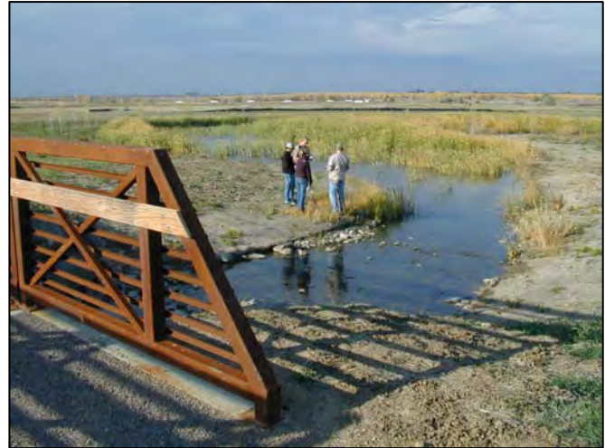
Cottonwood Creek after completion of Phase 2 – Choke point forcing floods to spill into the floodplain, providing pollutant reduction.
