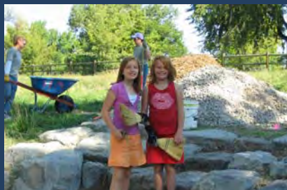
Student volunteers at a Denver trail building project
