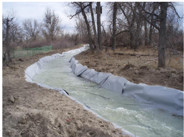
Photo 2 – Water Diversion Channel
