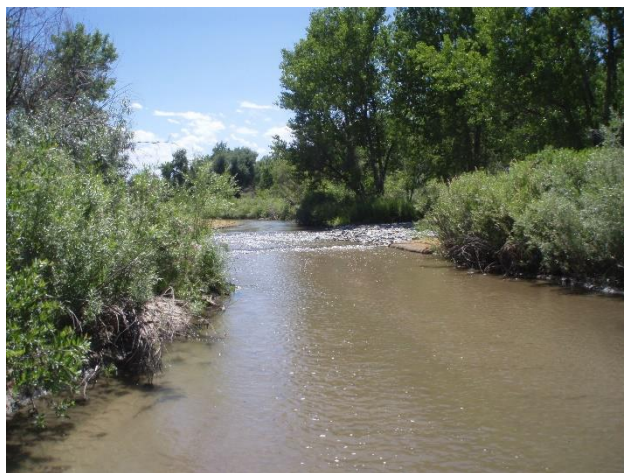
Photo 5 Constructed Void Filled Rip-Rap Drop
