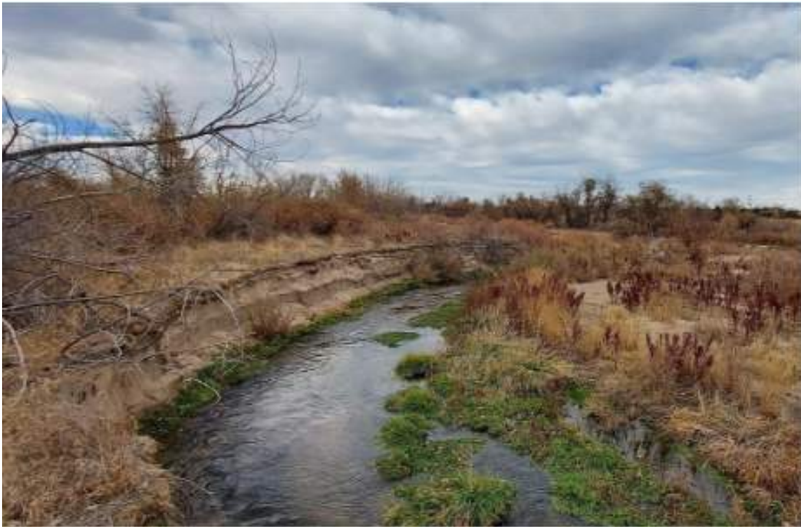
Figure 2: Bank Erosion Downstream of Arapahoe Road
