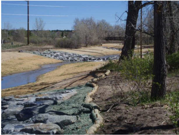
Photo 6 – Boulder Drop Structure Construction
