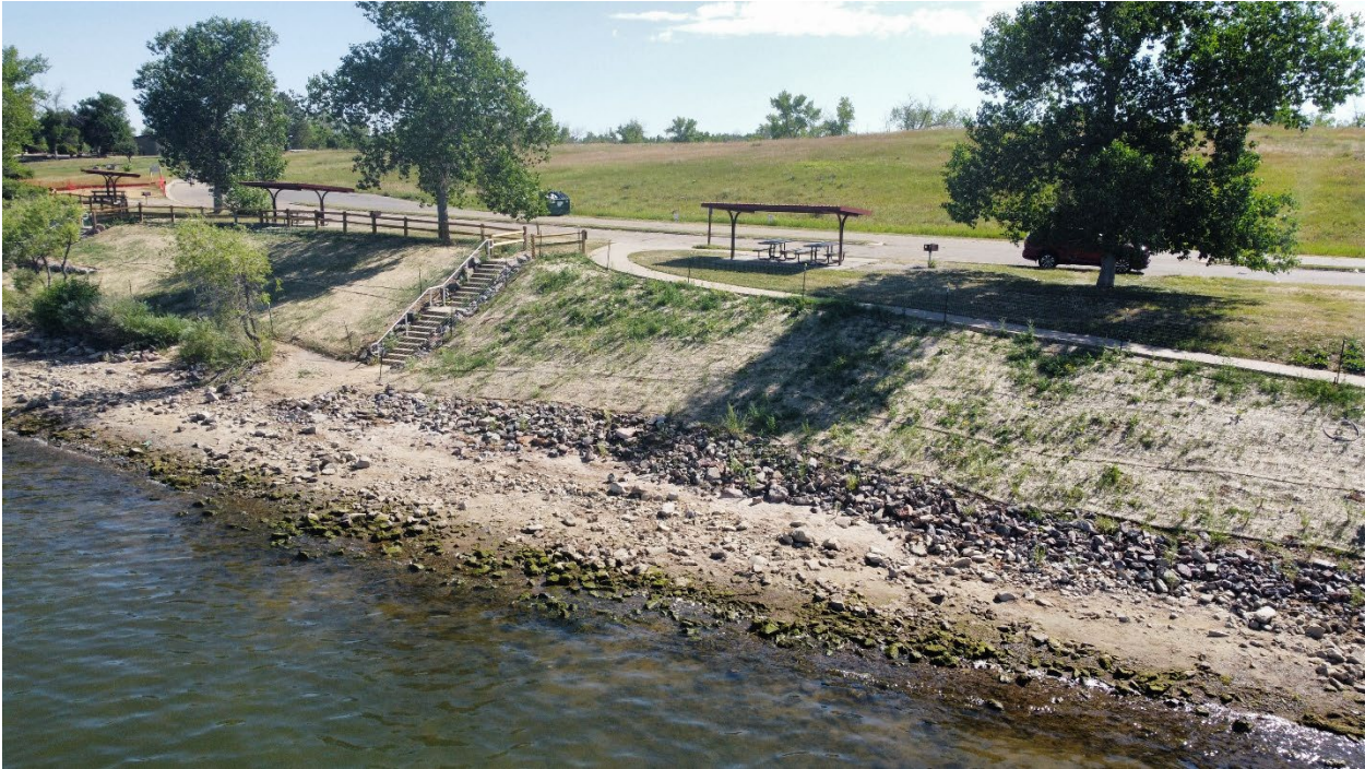
Figure 6: East Shade Shelter Project South Bank - Post Project
