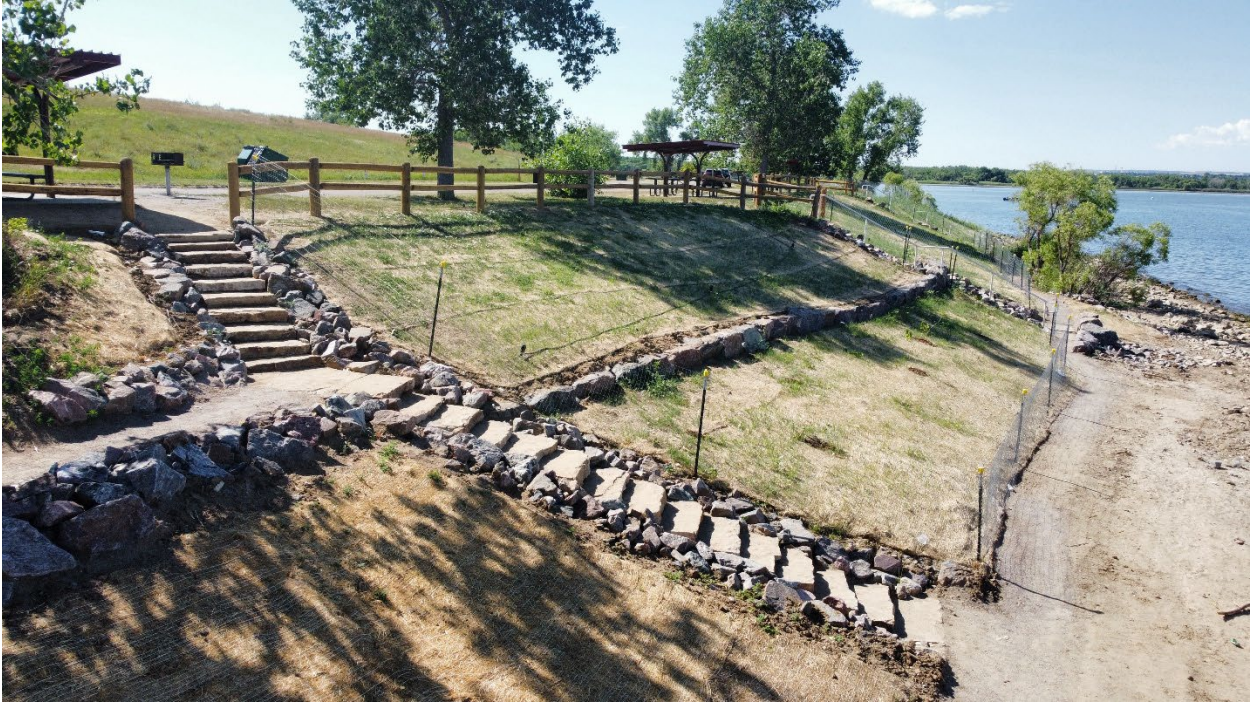
Figure 8: East Shade Shelter Project at North Staircase Looking South - Post Project
