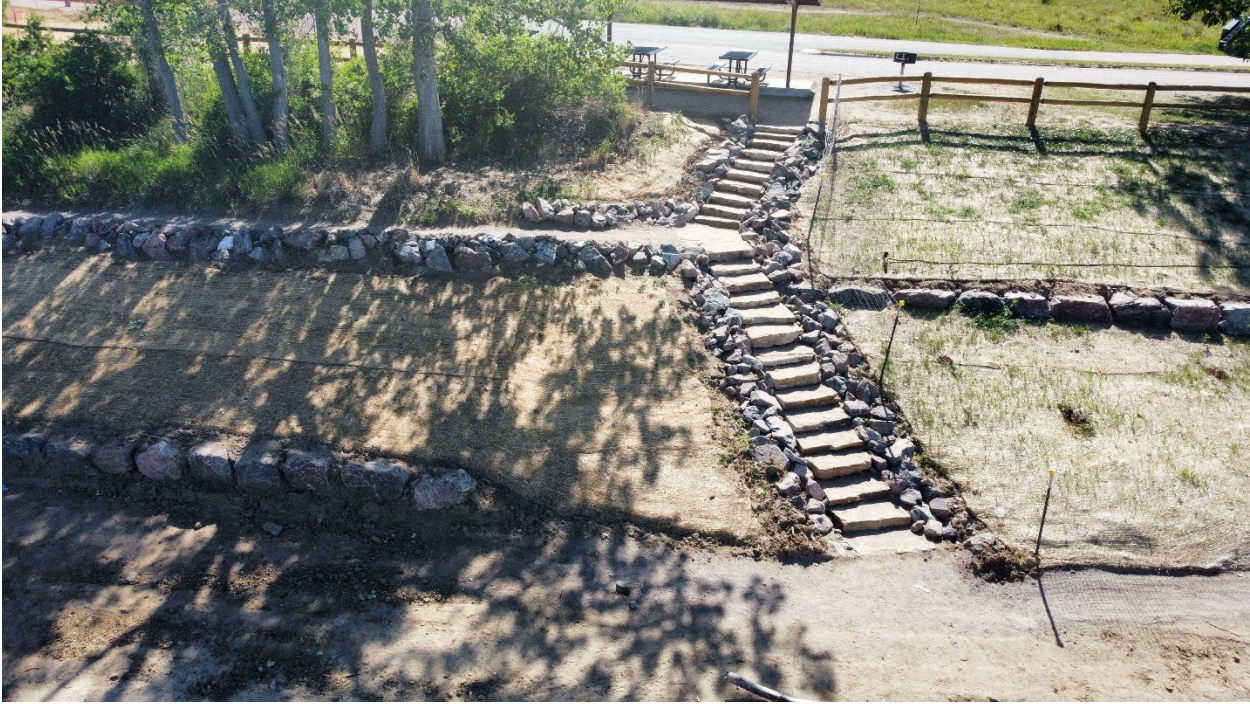
Figure 7: East Shade Shelter Project at North Staircase
