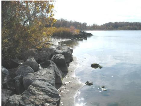
The boulder sizes exceed rock sizes needed to protect the shoreline from wave erosion. However, it was observed during some winter and early spring periods that ice forces were able to move and displace some large boulders at the east shoreline projects and, for
